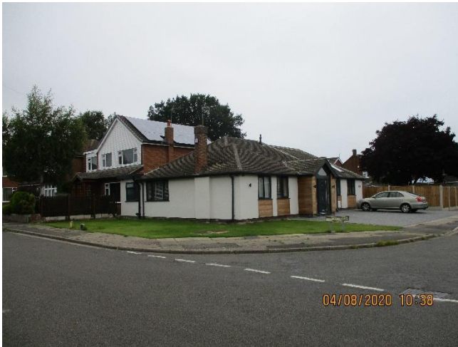
Front (south east) and side (south west) elevations viewed from Rivergreen Crescent.
