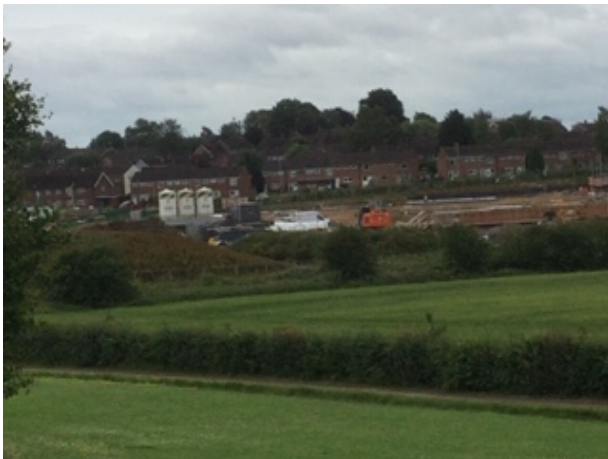
Phase 1 site from Pit Lane recreation ground with Ilkeston Road in background
